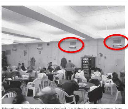
Tuberculosis Ultraviolet Shelter Study New York City shelter in a church basement. Note the ultraviolet germicidal irradiation fixtures located on the upper wall, directly below the vents. Photo: ©Randall Perry Photography.
